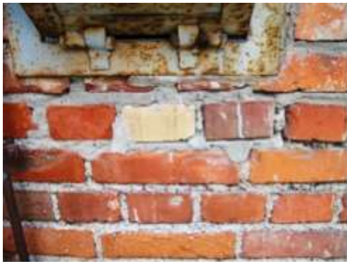
Photo 18: Mortar variation in right chute.
